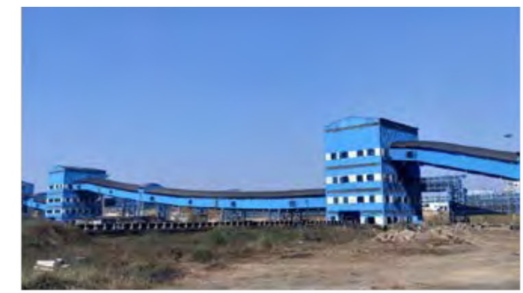
CHP NTPC Darlipali – 2X800 MW
