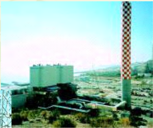
2 x 120 MW Steam Generators, Vasilikos Power Plant Unit I & II at Cyprus
