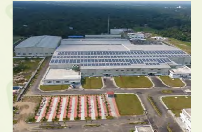
Food Processing Facility- ITC Panchla
