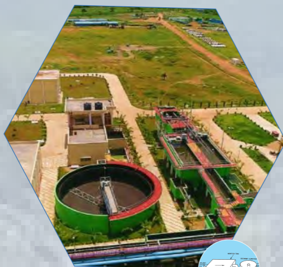
Constructing 43.5 MLD Sewage Treatment Plant in Odisha (WATCO)
