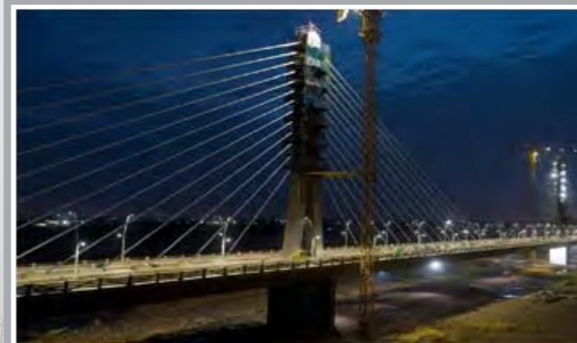
Karimnagar Cable Stayed Bridge
