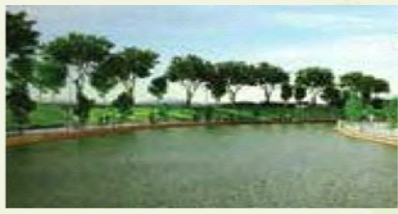
Rejuvenation of Amanishah Nallah (Dravyavati River), Jaipur, Rajasthan
