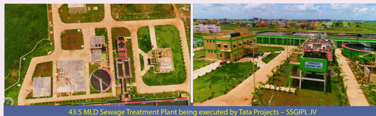
43.5 MLD Sewerage Treatment Plant being executed by Tata Projects – SSGIPL JV
