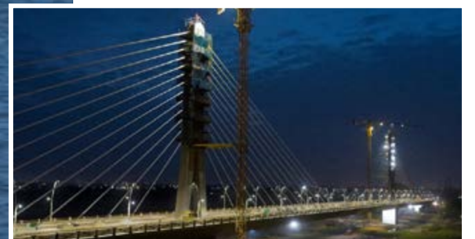
Karimnagar Cable Stayed Bridge
