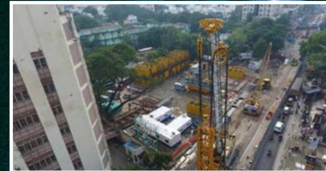
Trench Cutter for Diaphragm Wall Excavation
