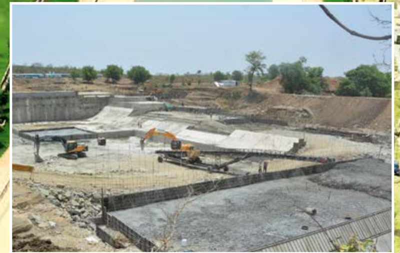
Concrete Dam Construction, Banda
