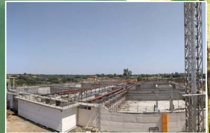
MLD Sewerage Treatment Plant, Ujjain
