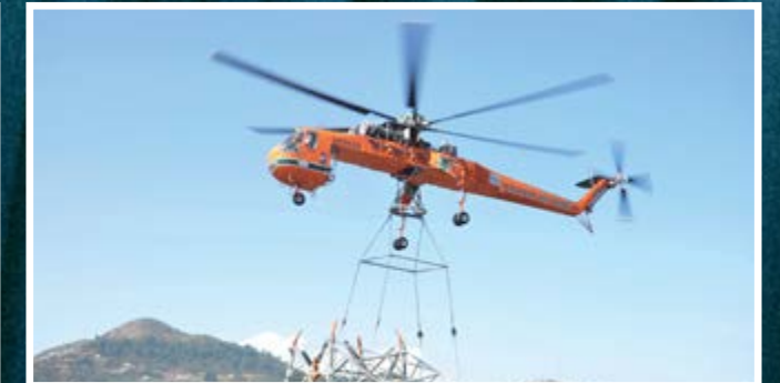
Tower Erection using Heli Crane
