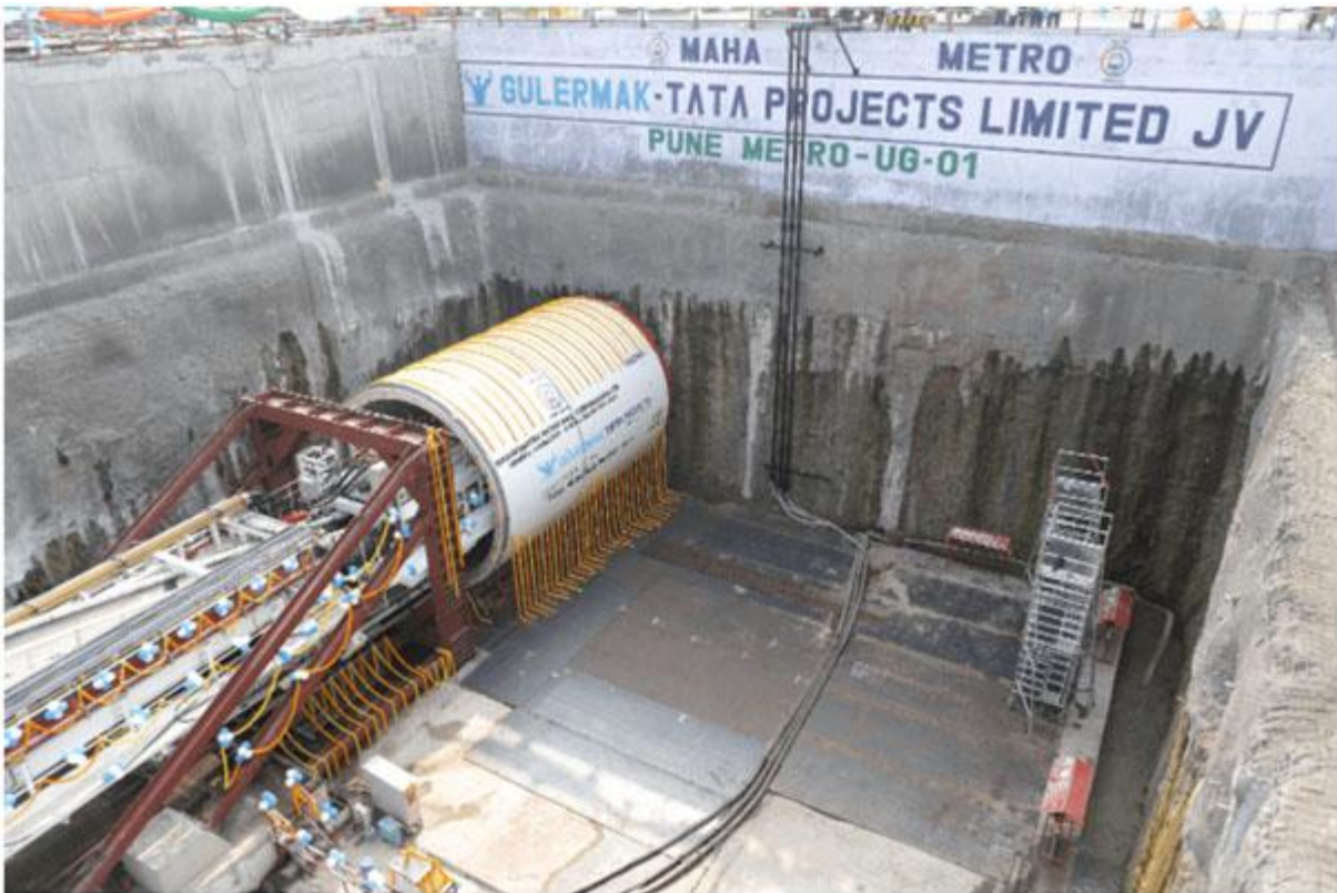
Pic: The approximately 279 feet long Tunnel Boring Machine that commenced work
