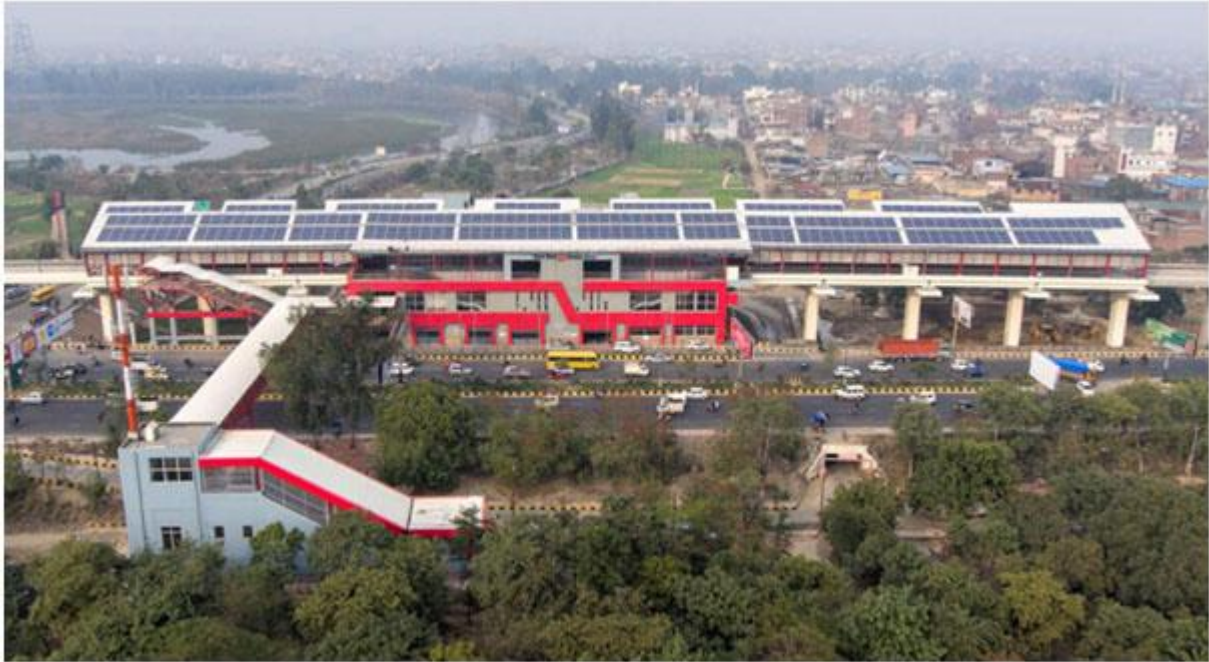
Pic: Hindon River Metro Station
