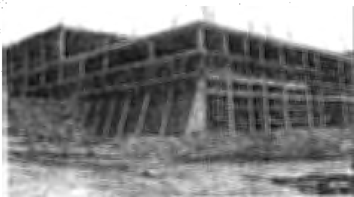
Polyester X-Ray Project, Ootacamund, under construction
