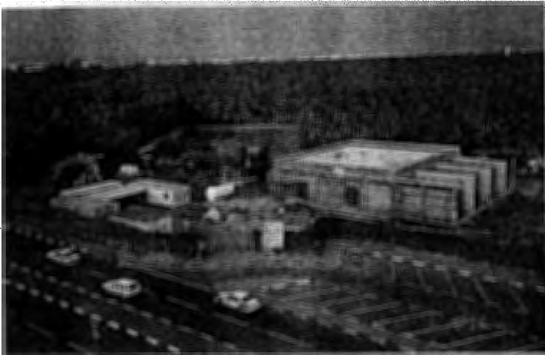
Reinforcement of 33 KV Network in Abu Dhabi and Al Ain, UAE—Town Centre Sub Station.
