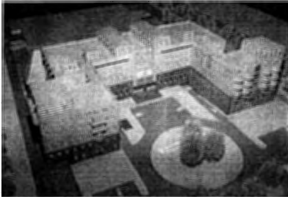
Model of Kalanidhi and Kalakosha Buildings of Indira Gandhi National Centre for the Arts at New Delhi
