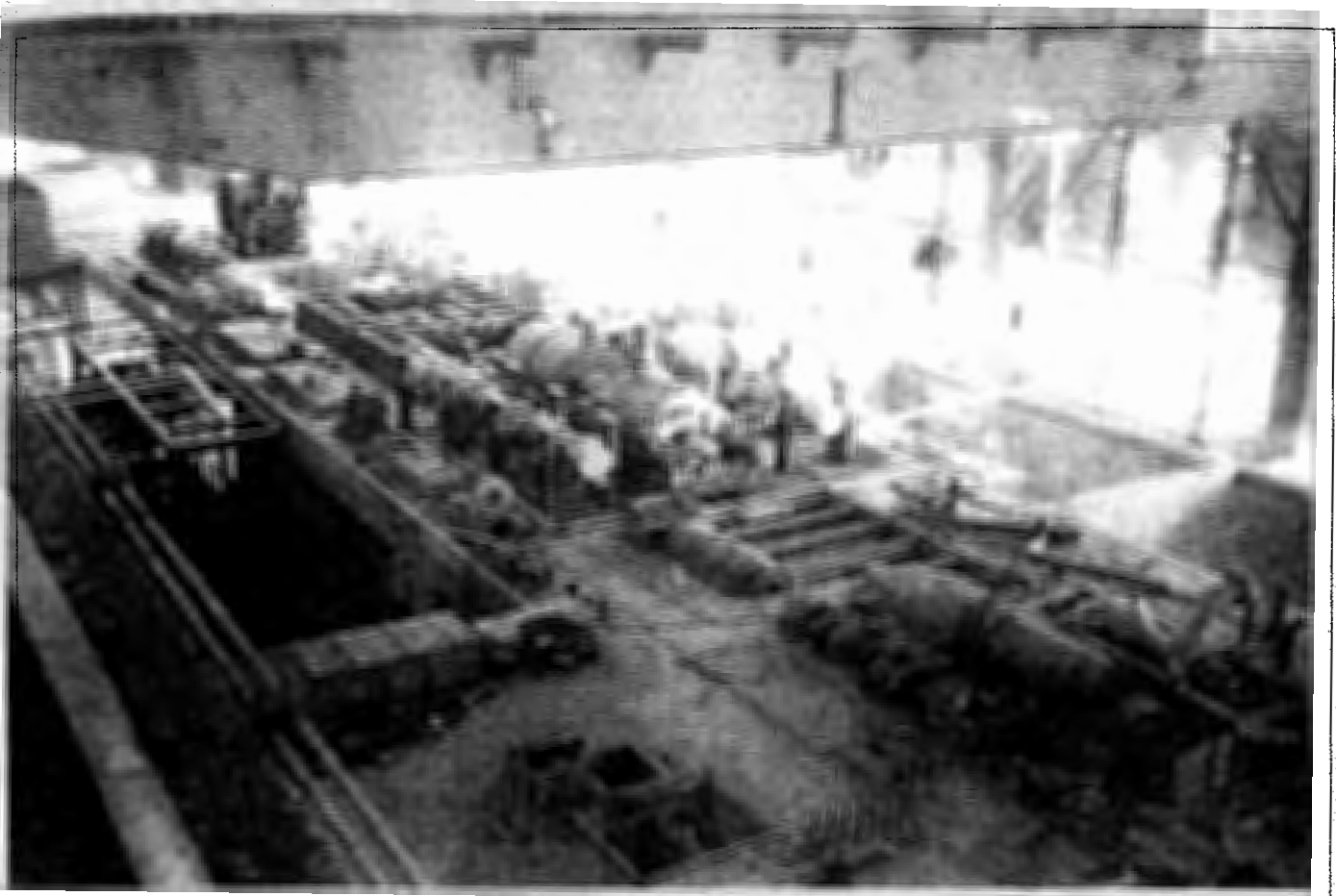
Erection—2 x 500 MW Turbo Generators at Rihand
