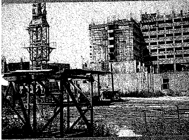
Hotel Project—Skeletal Frame—Construction
