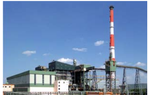
BoP for 2 x 77 MW CPP for HZL Chanderia
