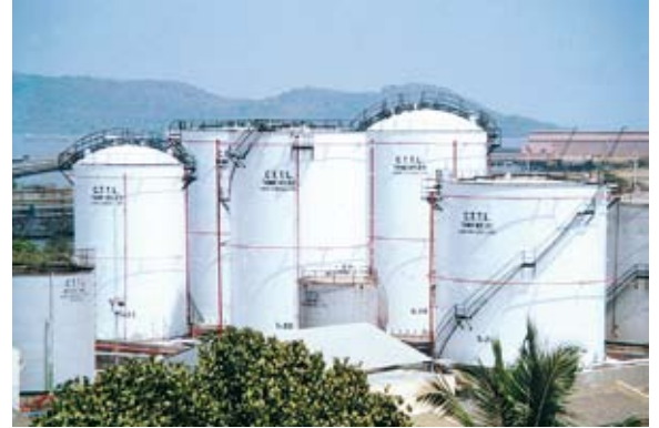
Oil Tank Farm, CCTL, Mumbai
