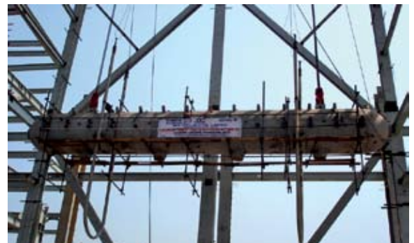
Erection of boiler pkg for 4 x 135 MW CPP for SEPCO Kharsuguda
