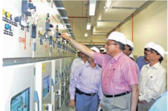
Switching on of GIS, 11 kV Substation, Pearl Island Project, Qatar
