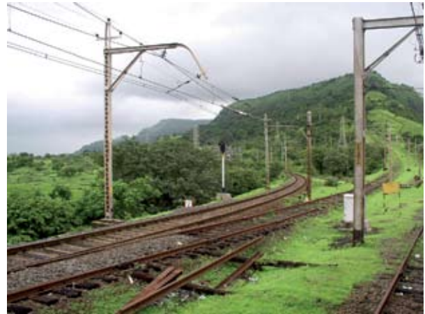
Railway Electrification Project, Central railway
