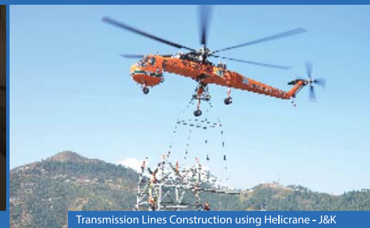
Transmission Lines Construction using Helicrane - J&K
