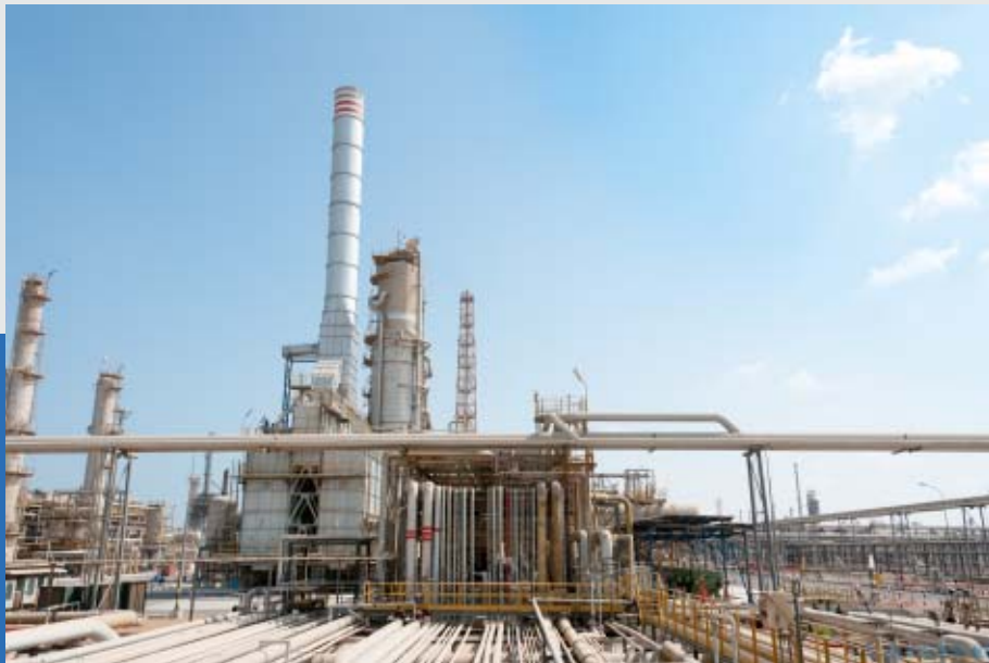
The cover visual depicts safe routing of safety valve at Ruwais and TAKREER Abu Dhabi Refinery Project, Abu Dhabi, UAE
