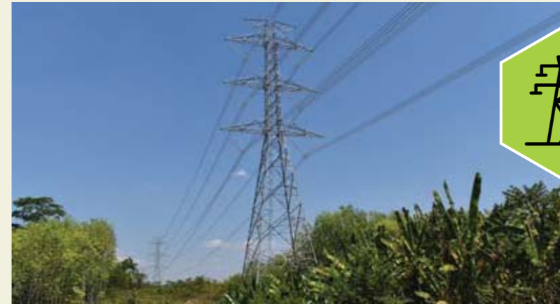
Completed 41.42-km Transmission Line Project of 500 kV in Thailand
