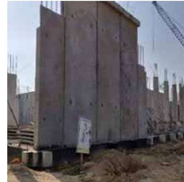
Precast Technique Without End Bearings/Bracket/Sleeves
