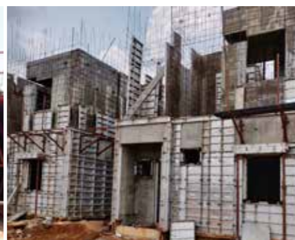
Alternate Materials - Using Aluminium Formwork Instead of Wooden Shuttering
