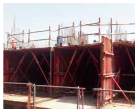
Alternate materials - Using Tunnel Formwork Instead of Conventional Formwork
