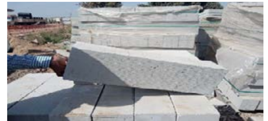
100% Alternate material used . AAC Blocks and Fly Ash Blocks are used
